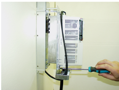
Installing the bottom cover to the back plate (frame size D only)
