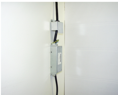
Mounting the assembled unit with RFI-filter
